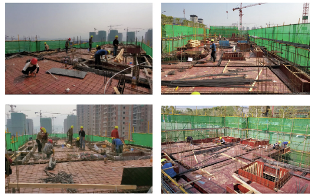
Fig. 8. Video frames of the construction scene.
