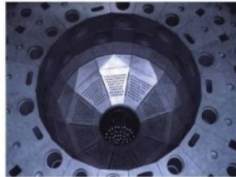
Second generation nuclear graphite Representative products: IG-110 (used in HTR-10 and HTTR) H451 (planned to be used in the gas-cooled reactor in US) ATR-2E (planned to be used in the gas-cooled reactor in Germany)
