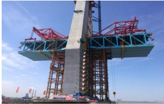
**Fig. 8.** Hoisting of double section Hutong Yangtze River Bridge girder.
