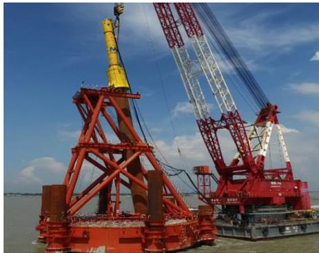
Fig. 4. Steel pile inserted by a fixed guide frame.
