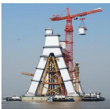
Fig. 6. Large-scale tower crane lifting a subsection.
