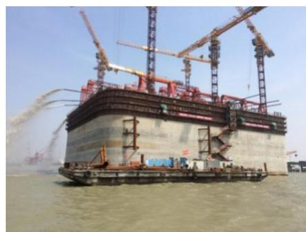
**Fig. 3.** Upper concrete caisson.
