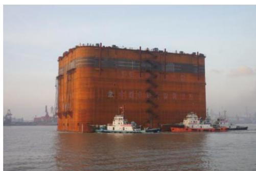
**Fig. 2.** Floating transportation of steel caissons.
