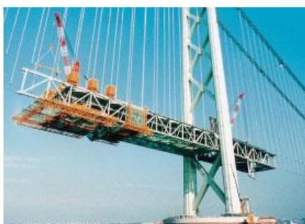
Fig. 10. Girder chip by girder crane.
