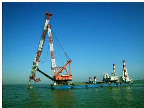
Fig. 5. Steel pile inserted by a barge.
