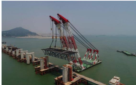
**Fig. 9.** 80 m full-span hoisting of the Pingtan Railway Bridge.
