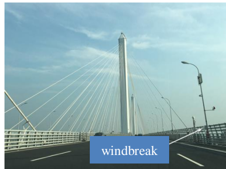
Fig. 5. The windbreak at Jiashao Bridge.
