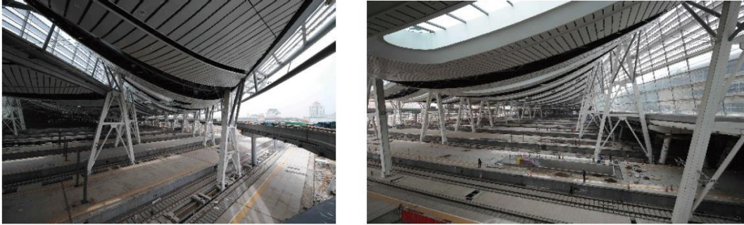
Fig. 3. Beijing South railway station during construction.
