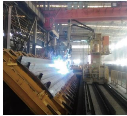
(b) Welding robot for steel bridge deck plate
