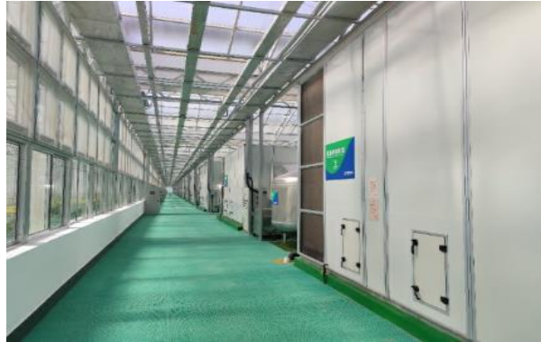
Fig. 2. Greenhouse environment integrated control system based on positive pressure ventilation.
