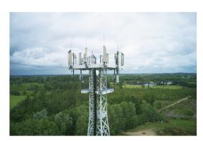
**Fig. 1.** 5G towers like this one are now transmitting at frequencies that are close to the frequencies used by aircraft altimeters. Expanding service to these frequencies offers better performance for cell phone users but could interfere with the proper functioning of some altimeters. Credit: Fabian Horst (CC BY-SA 4.0).
