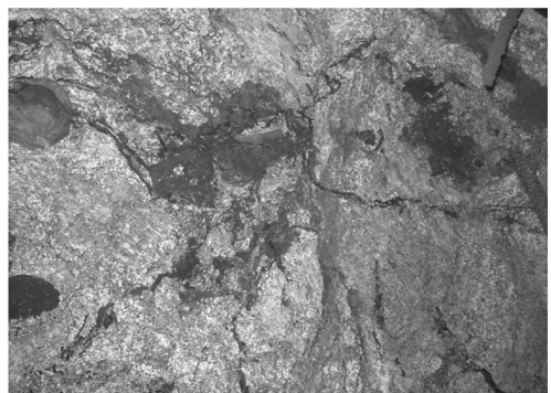
图4 开挖面浆液扩散情况 Fig.4 Grout diffusion at excavation face
