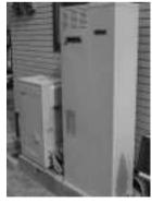
图7 利用 Kyocera 阳极支撑扁管电池制造的700 W SOFC CHP 单元(左:SOFC 系统;右:热水箱) Fig.7 A 700 W SOFC CHP unit (left: SOFC system; right: hot water tank) utilizing Kyocera's anode-supported flat tubular cells
