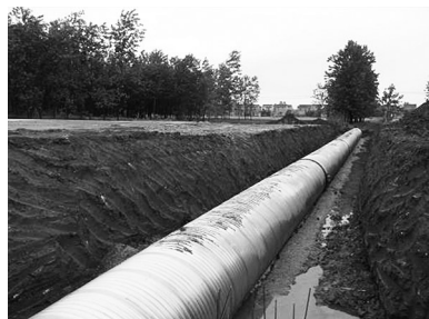
图1 K14+176.4螺旋形整体栓接钢波纹管 Fig.1 The spiral and whole bolting steel corrugated pipe in K14+176.4
