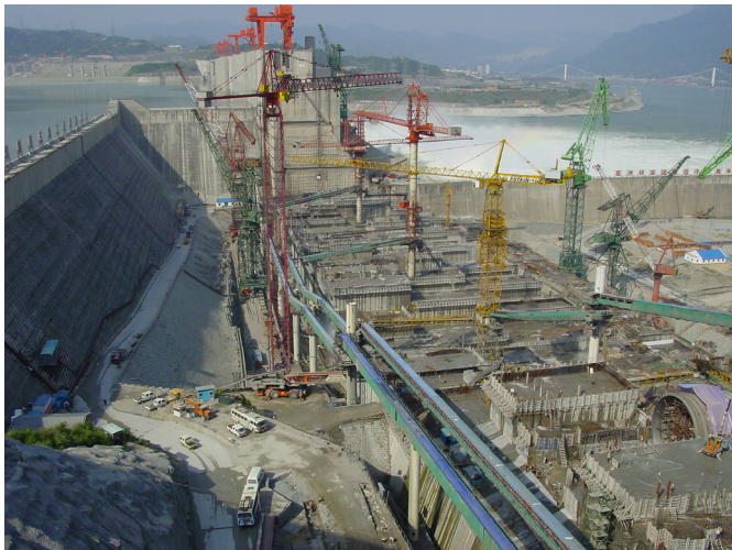
Figure 2. Construction site of the Phase III Dam.
