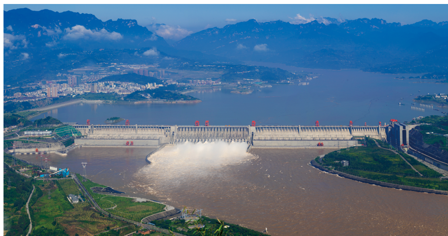
Figure 1. The completed Three Gorges Hydro Junction Project (2014, Zhengping Huang).
