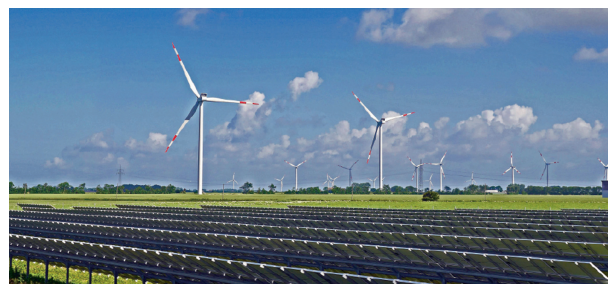
Fig. 1. International green hydrogen projects plan to build dual renewable energy plants to power electrolysis. For example, the Asian Renewable Energy Hub in Western Australia, shown here in an artist's illustration, will have a photovoltaic farm to harvest solar energy during the day and nearby wind turbines to collect energy during windy nights. Combining renewable power sources maintains the energy needed for green hydrogen production, without relying on fossil fuels. Credit: Pixnio (CC0).
