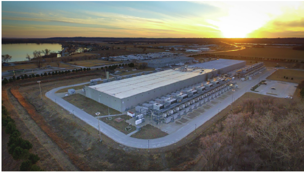
Fig. 2. Large, cloud-accessed data centers like this one built and operated by Google in Council Bluffs, IA, USA, can draw more than 100 MW at any given time—consuming roughly as much electricity as 80 000 homes—and have cooling systems that can guzzle up to 3 \times 10^9 L of water a year. Google claims that all its data centers will be running entirely on renewable energy by 2030. Credit: Chad Davis (CC BY 2.0).
