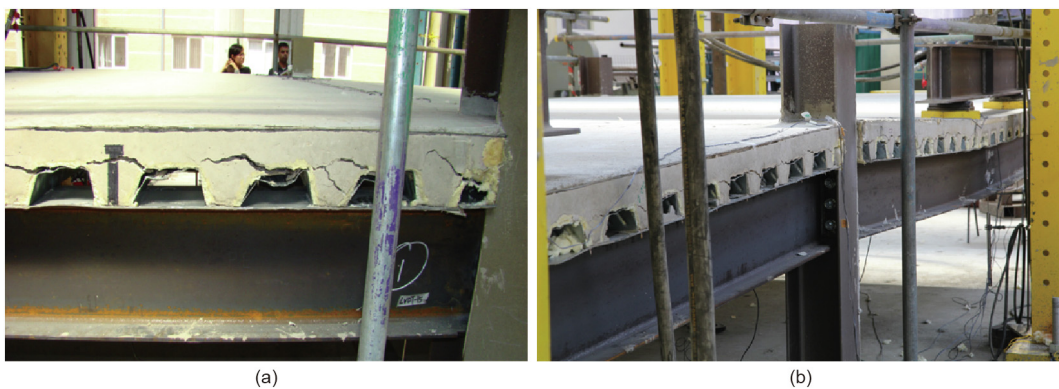
Fig. 19. (a) Crack at the edge of the slab without U-bars at failure, and (b) deflection of the edge beam with U-bars.
