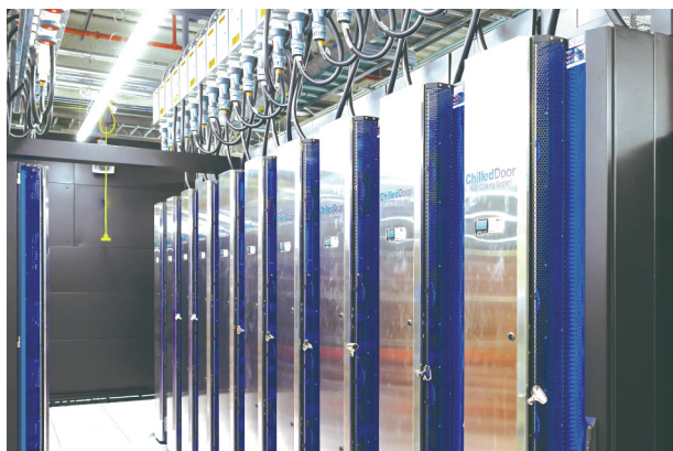
Fig. 2. Part of Frontier’s cooling system, which can circulate more than 151 000 L of water per minute through the machine. The system is 30%–40% more efficient than the cooling system of its predecessor supercomputer, Summit. Credit: Oak Ridge National Laboratory (CC BY 2.0).
