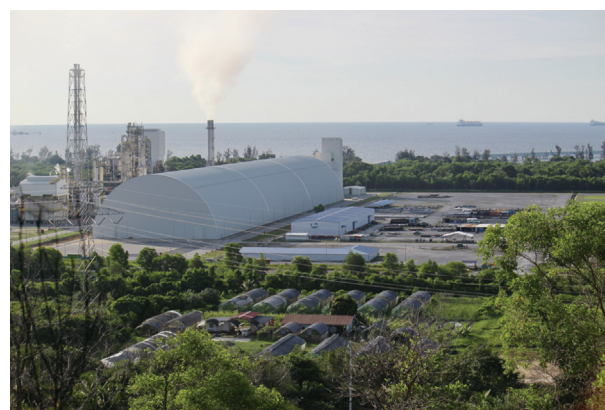
Fig. 2. Like almost every other ammonia plant in the world, this one in Brunei burns fossil fuels to produce ammonia via the Haber–Bosch process. The facility, which opened in 2022, produces 2200 tonnes of ammonia daily. Credit: DeltaSquad833, Wikimedia Commons (CC BY-SA 4.0).
