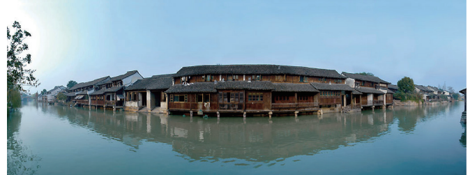
Fig. 8. Many small Chinese towns have retained their cultural characteristics. Available from: http://www.wuzhen.com.cn/cn/tupian.aspx?cid=88 .
