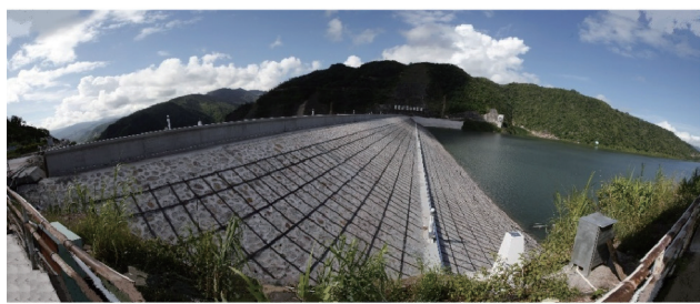
Fig. 9. New anti-seismic measures taken for the Nuozhadu earth core rockfill dam.
