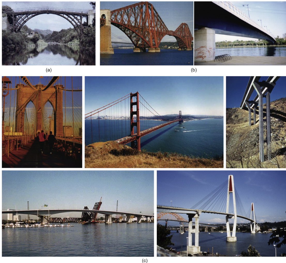
Fig. 2. The introduction of steel stimulated the development of new bridge forms. (a) Iron did not change the bridge form much (Coalbrookdale Iron Bridge by Pritchard); (b) high-strength steel wires stimulated new bridge types; (c) after high-strength steel wires became available, bridge construction started a brand new chapter.
