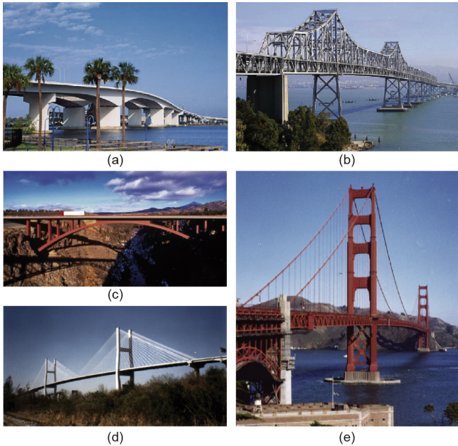
Fig. 3. Bridge types. (a) Acosta Bridge (girder); (b) Old San Francisco-Oakland Bay Bridge (truss); (c) Crooked River Bridge (arch); (d) Talmadge Memorial Bridge (cable-stayed); (e) Golden Gate Bridge (suspension).
