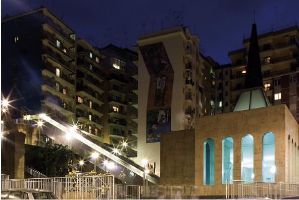
Fig. 1. Salvator Rosa Station. (Photo credit: Luca Pioltelli)
