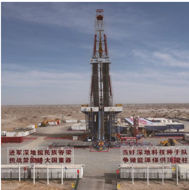
Fig. 11. The 12 000 m drilling rig for the SDTK #1 Well.
