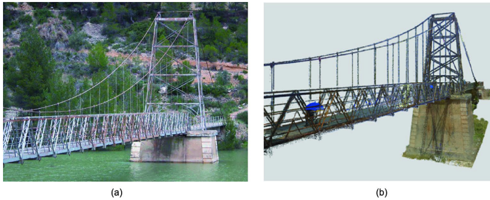
Fig. 6. Pajareles footbridge. (a) Photograph of the structure; (b) point cloud visualization.
