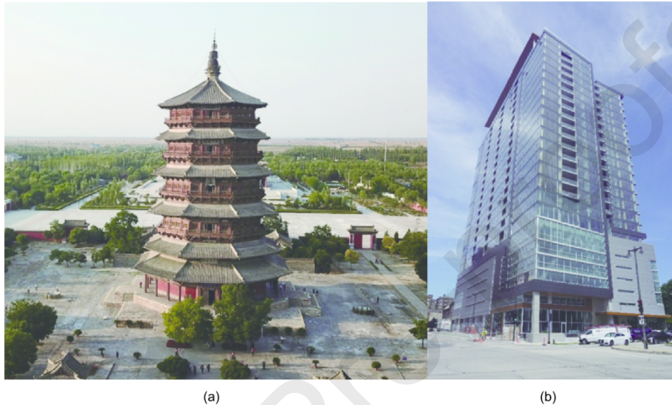
Fig. 2. (a) The Sakyamuni Pagoda of Fogong Temple in Yingxian, Shanxi, China, which is more than 67 m tall, was built entirely from wood and completed in 1056. (b) The Ascent MKE in Milwaukee, WI, USA, completed in 2022, is the world’s tallest mass timber structure with a height of 87 m. Credit: (a) Charlie Fong/Wikimedia (CC BY-SA 4.0); (b) Michael Barera/Wikimedia (CC BY-SA 4.0).
