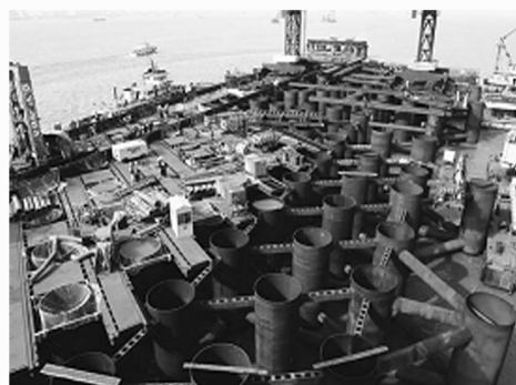
Fig.2 Establishment of north and south pylon foundations construction platform
