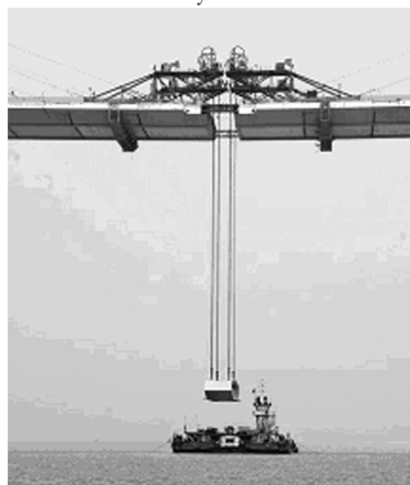
Fig. 4 Girder erection for middle span closure
